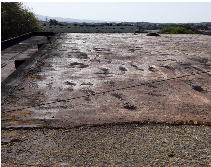
Photograph showing removal of existing waterproofing membrane/medium on the Regional Office roof.
