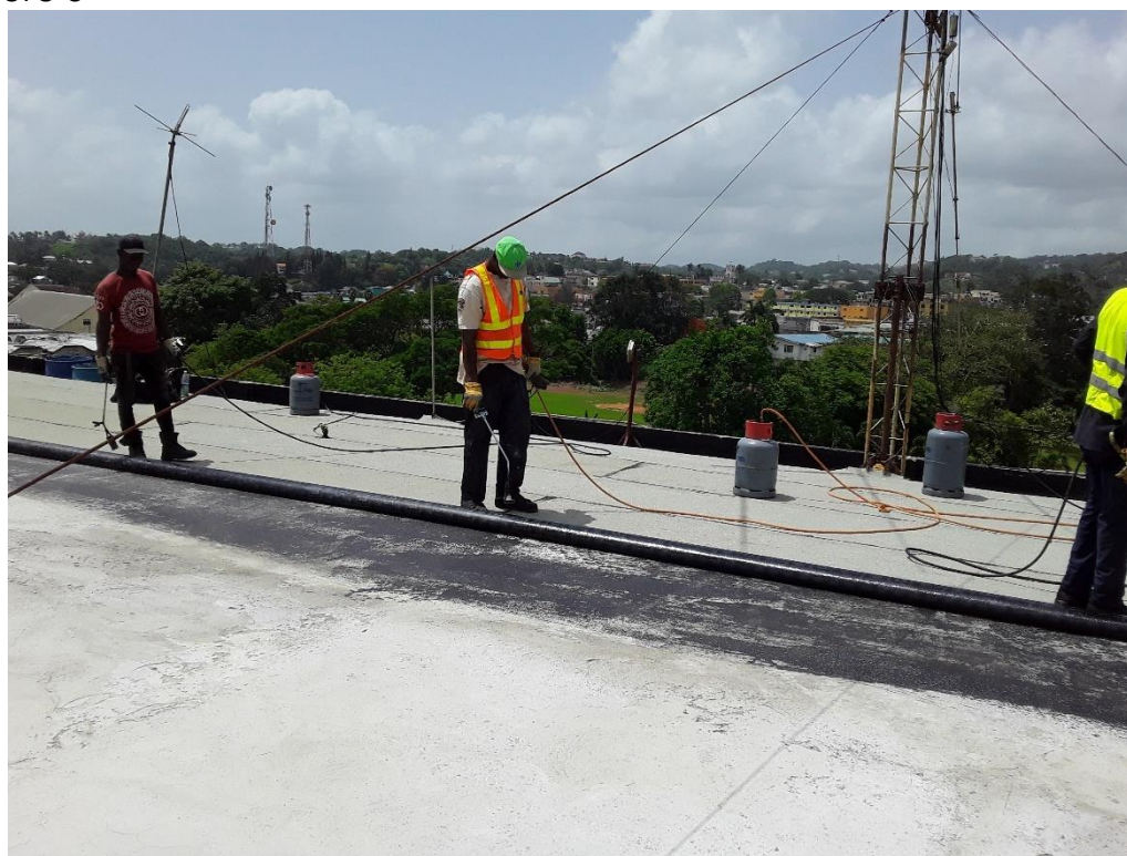
Installation of waterproofing membrane, including primer.
